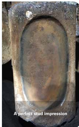
Very low corrosion impact, perfect stud placement, no loose studs and consistent and satisfactory measurements of link dimensions is the result from the inspection.
